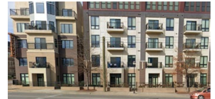
Individual entrances to ground floor apartment units, source: Google Street View
