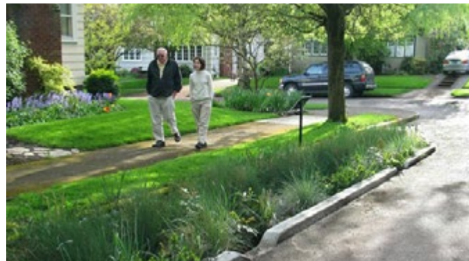
Example of a bioswale along a neighborhood street, source: ASLA
