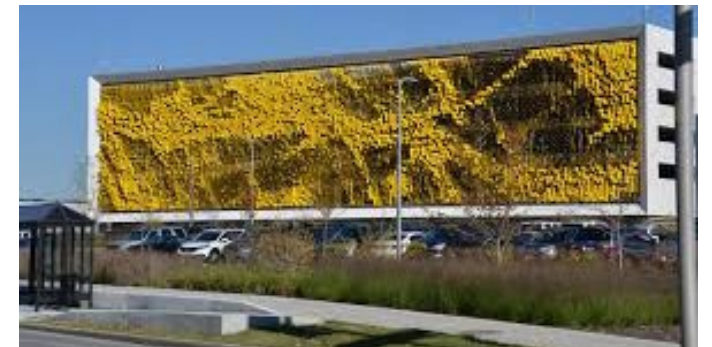
Parking structure with integrated public art, New Eskenazi Replacement Hospital, source RG Collaborative
